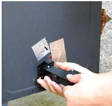
Figure 4. Insert the spring to the hole
